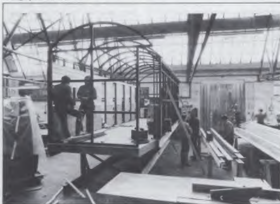
The train under construction at Kimpian Walker Ltd in Brixton. Photograph: David Watson.
